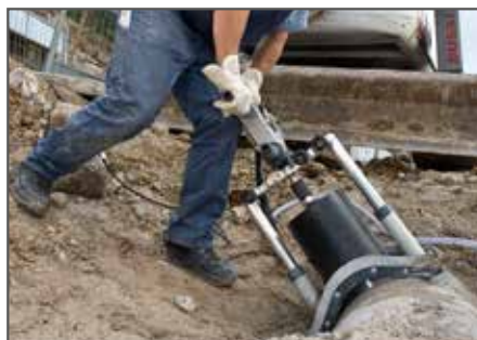
Wet drilling in a concrete pipe, with BST drill stand
