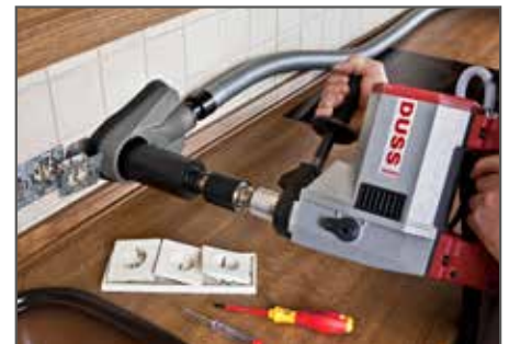
Clean wet drilling in concrete with DUSS suction cup, hand-held
