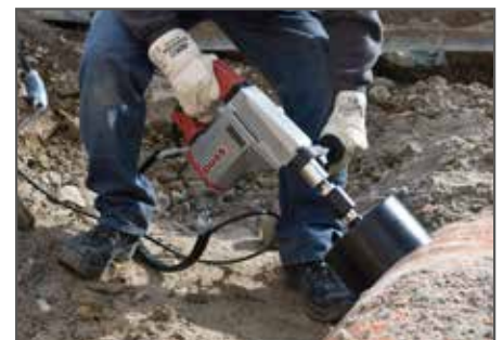
Dry drilling in a plastic pipe, hand-held
