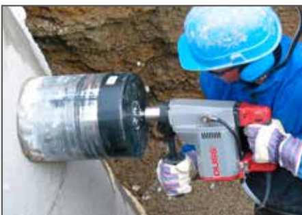
Wet drilling in a concrete shaft, hand-held
