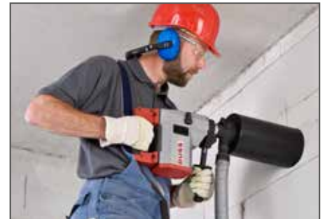
Dry drilling in masonry with dust extraction, hand-held
