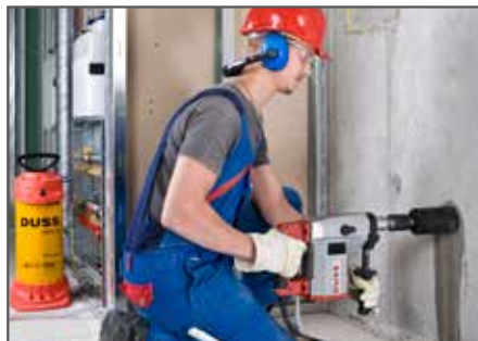
Electrical socket sinking in concrete – wet, hand-held
